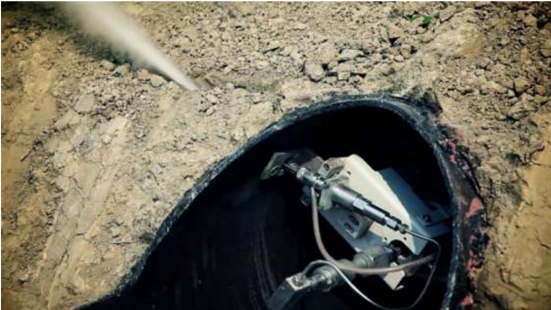
Figure 9 (a-b)– Cutting phase during site tests
