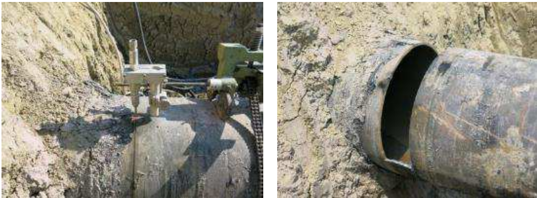
Figure 13 – Pipeline external cutting.
