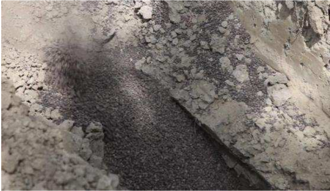
Figure 11 (a-b-c) – Filling phase with expanded clay during site tests
