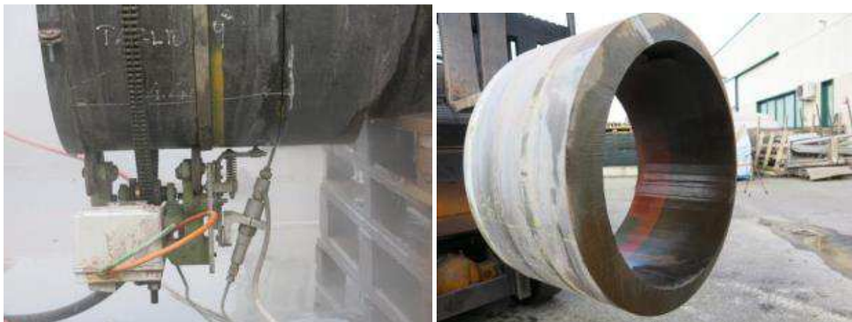
Figure 14 (a-b-c-d) – Beveling end on very high wall thickness steel pipes.
