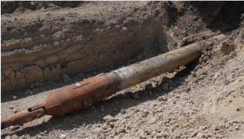
Figure 10 (a-b-c-d) – Extraction phase during site tests
